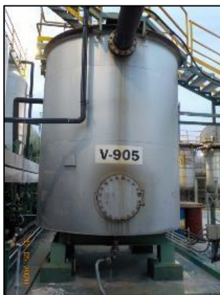
pH Control Tank (PC1)
